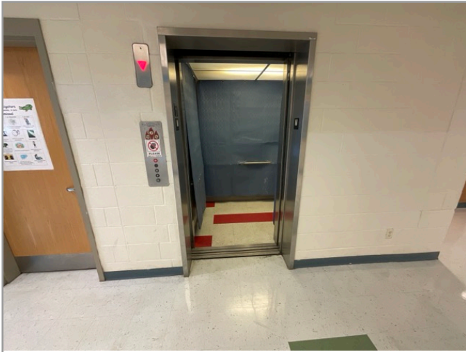
LOBBY LOOKING AT CABS
