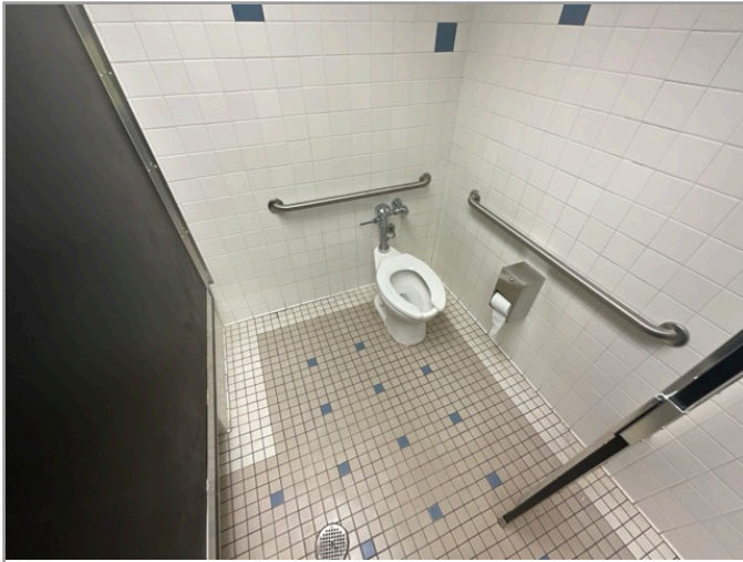
TOILET STALL OVERVIEW
